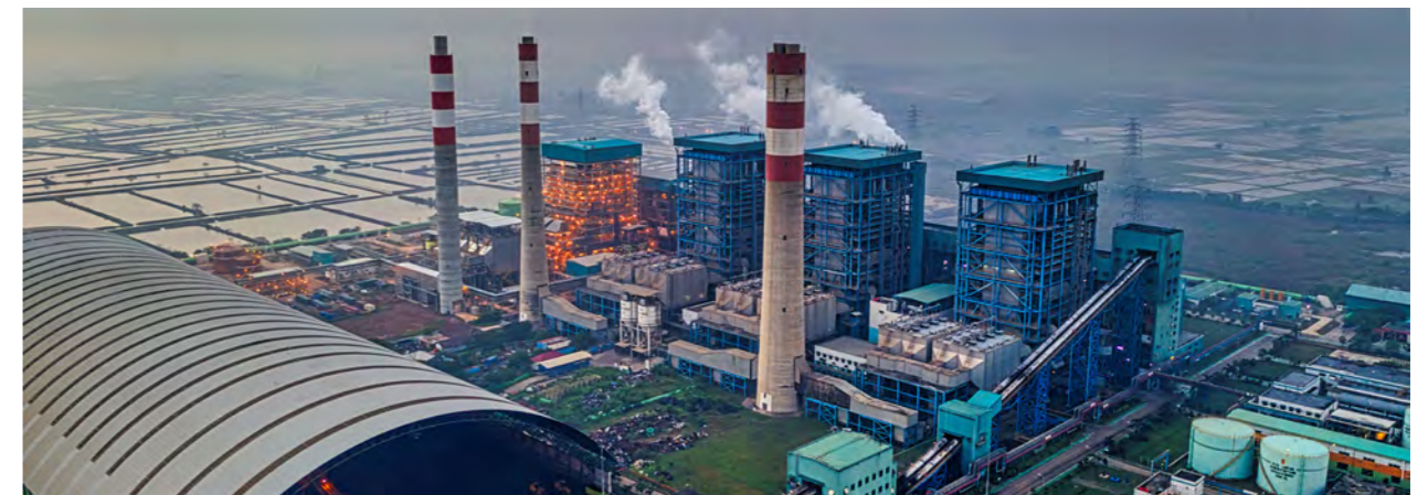
Industrial Equipment Pressurization
